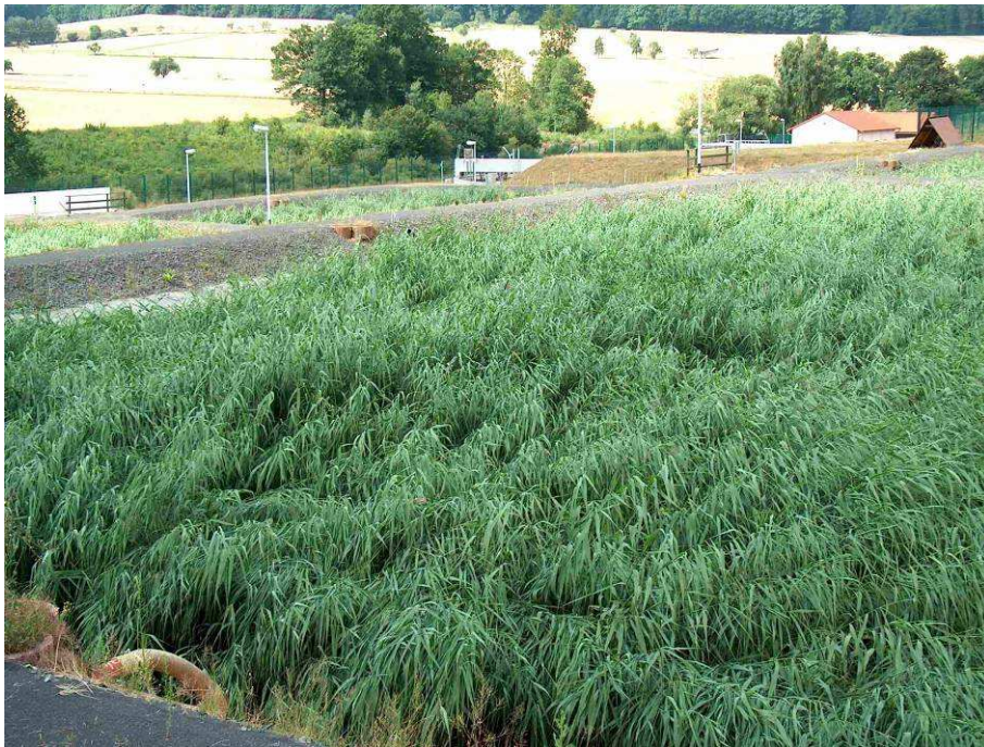
One of four reed beds at sewage treatment plant Bad Emstal (6,000 m 2 in total)
