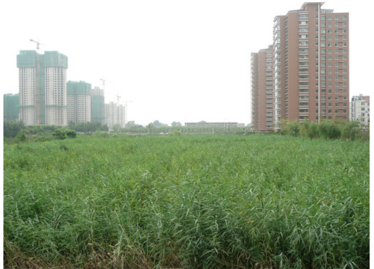
Reed bed treatment system
