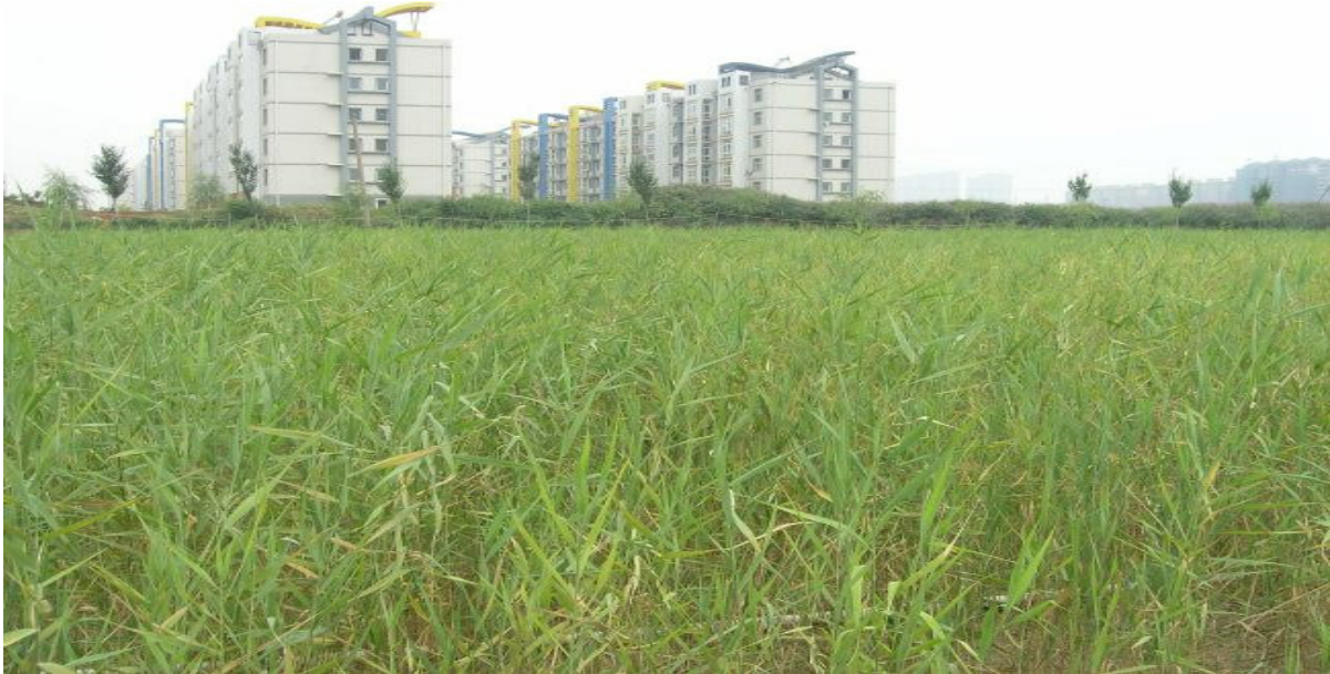
Municipal wastewater treatment plant in Shenyang China
